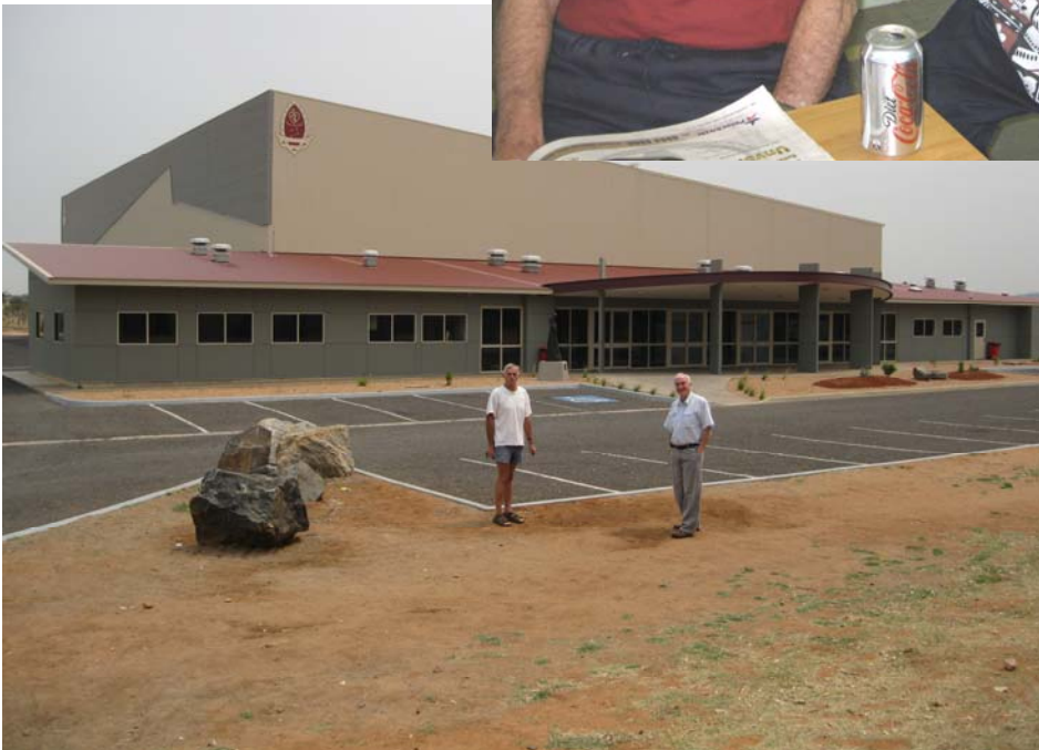
Brs Ron Campbell and Paul Gilchrist showing off the new Gym at OLSH.
