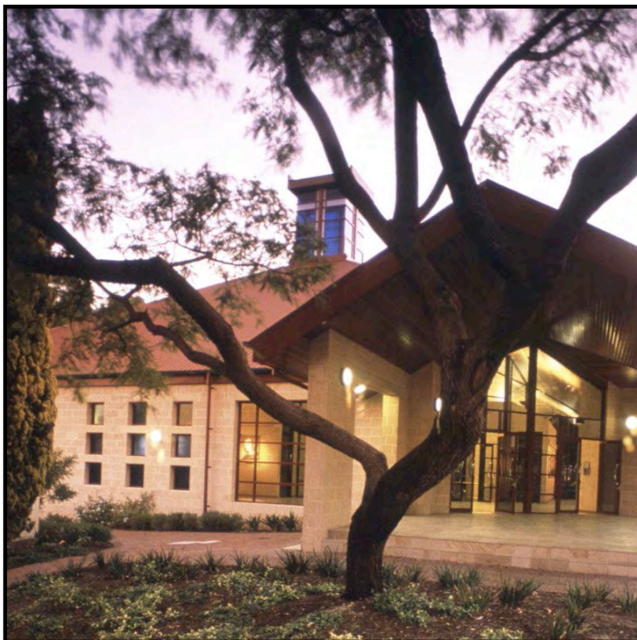
The Newman College Chapel, dedicated to St Marcellin Champagnat. Br Stephen’s last and crowning achievement as a builder.
