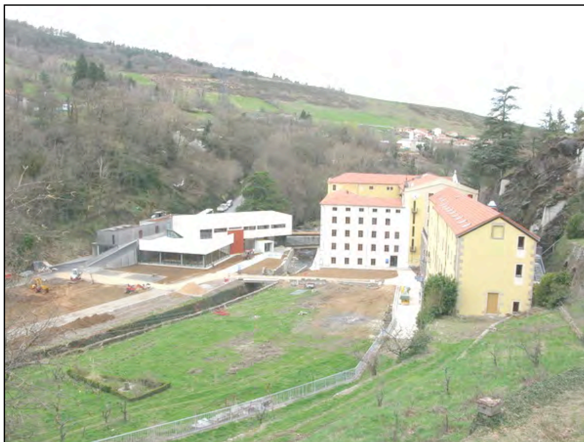
The renovated Hermitage nearing completion
